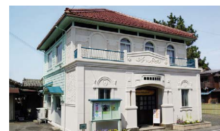
The former Kyoto Dento Takahama Sales Office, designated as a national registered tangible cultural property
